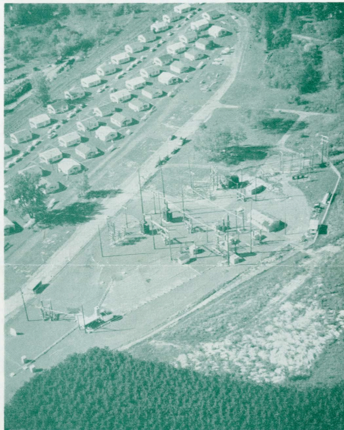
EHV Cable Testing Facility, Cornell University
