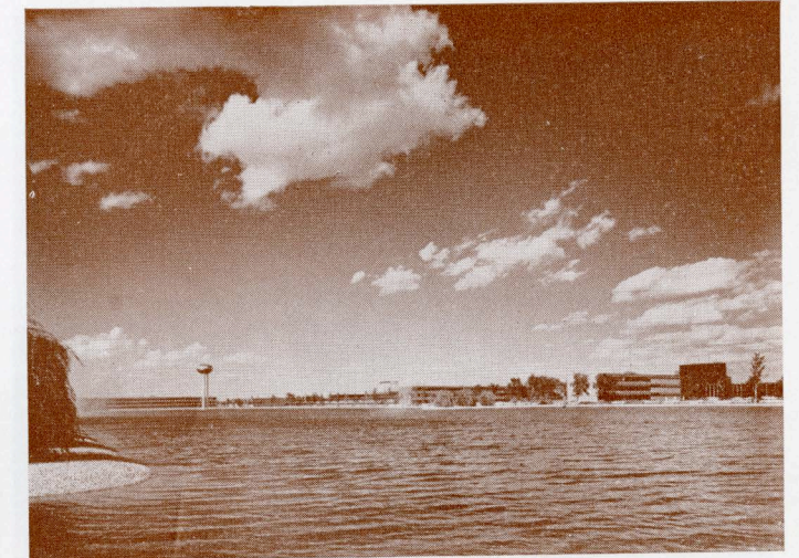
General Motors Technical Center
