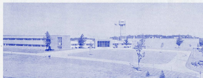
Pennsylvania Electric Co., Erie, Pennsylvania.
