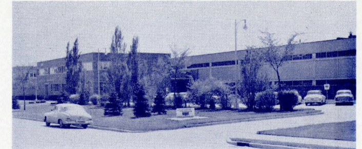
Cutler Hammer Northside Plant
