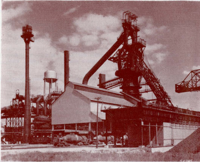
Modern Blast Furnace at Middletown Works Armco Steel Corp.
