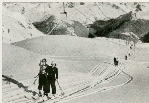
Huge span, 918 feet long
