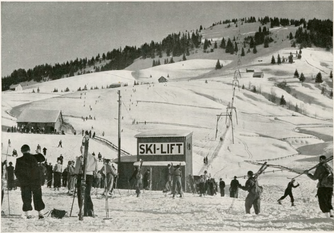
Length 3960, ascent 1360 feet, 10 pillars
