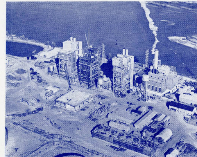
Construction Work at Tulsa Power Plant
