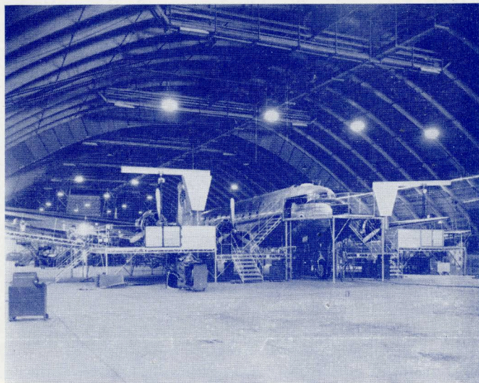
Northwest Airlines Overhaul Base, Hohman Field, St. Paul.
