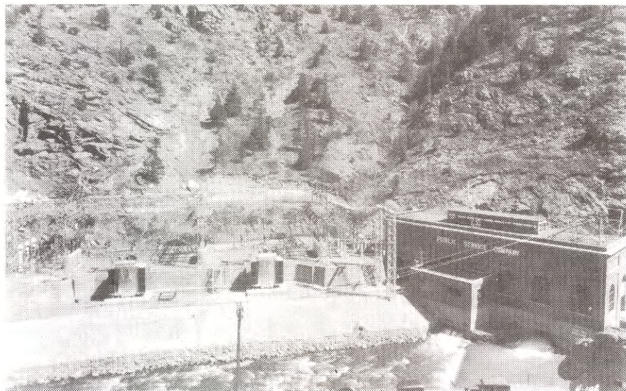
Figure 14. Boulder Canyon Hydroelectric Plant, constructed in 1906. Construction was suspended in 1907 due to a depression, but was completed in 1910. The capacity was 10,000 k.w. in two machines. It was rebuilt to a 20,000 k.w. capacity. The original indoor transformer was replaced with two outdoor units in a new substation on the left. A 44 k.v. substation was added to the right and off the photo.
