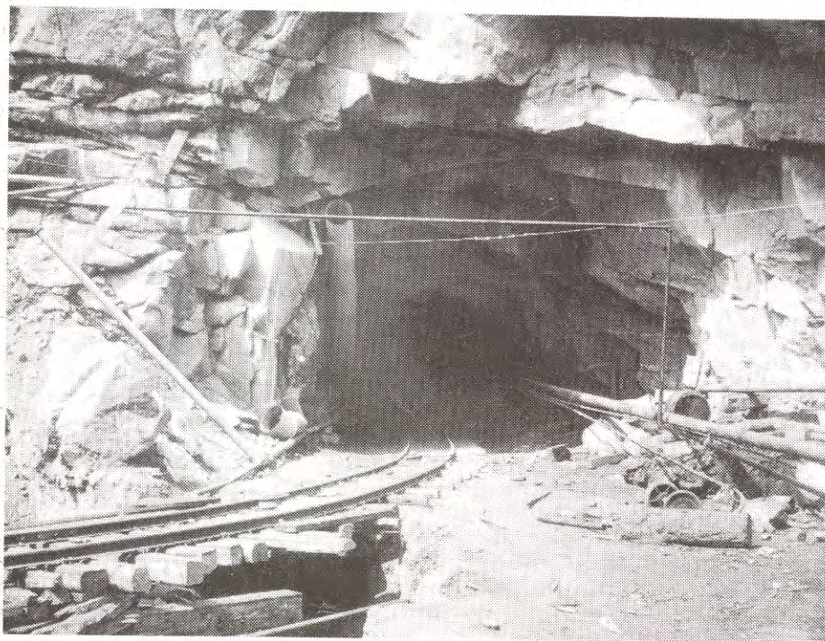
Figure 9. Diversion tunnel carrying water from the Colorado River to Shoshone hydroelectric plant. This tunnel is 2½ miles long and was bored through the granite wall of the canyon.
