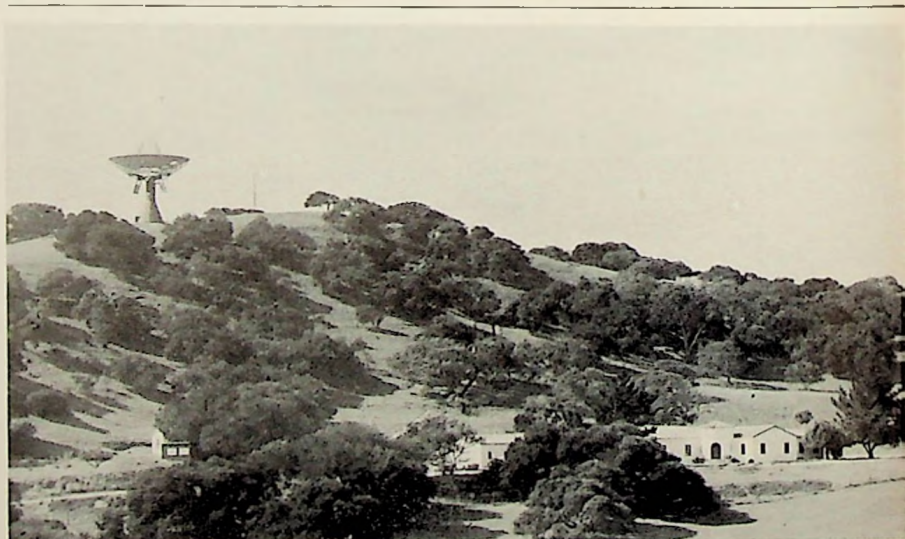
Nearing completion at Rancho Arroyo Seco just outside Monterey is a 60-ft parabolic antenna on an azimuth-elevation mount. It will be the first functioning element of the advanced engineering division of D. S. Kennedy Inc., formerly Satellite-Kennedy. The antenna and related facilities will be made available to outside organizations for propagation studies. Robert J. Grenzbeck, vice president for advanced engineering, will have charge of the antenna range. Howard H. Hubbard is chief engineer
