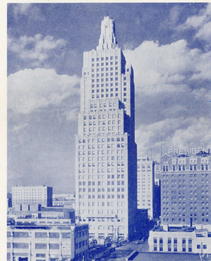
Kansas City Power and Light Co. Building
