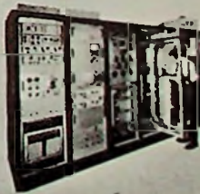
High Power Signal Source—ultra-stable 40 mc to 40 Gc system for electromagnetic compatibility and RFI measurements.
