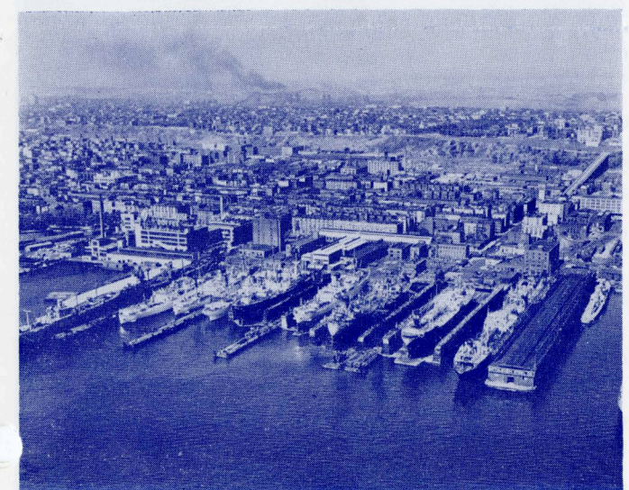
Hoboken Yard, Bethlehem Steel Co.
