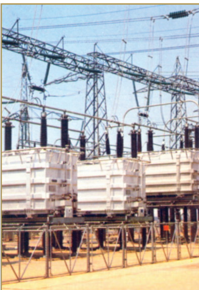
figure 10. An outdoor dead tank thyristor valve, Cabora-Bassa HVdc link; from BBC brochure CH-A-023 880 E (photo courtesy of ABB Asea Brown Boveri Ltd., Zürich, Switzerland).
