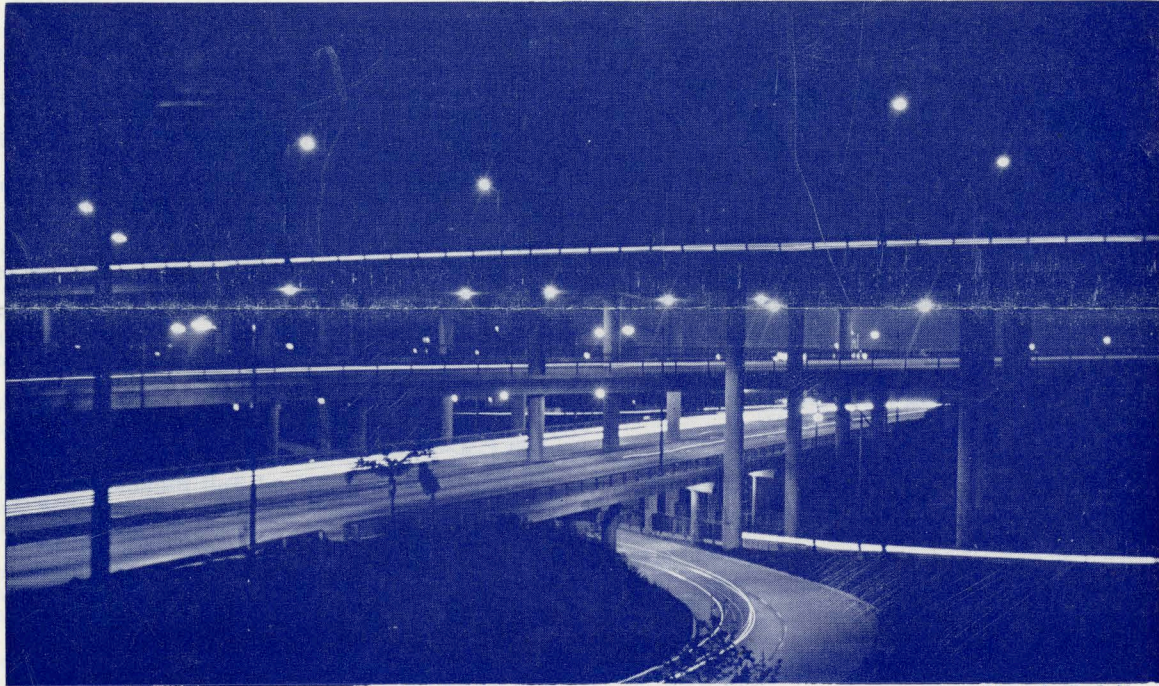
"The Stack," Los Angeles Freeway System
