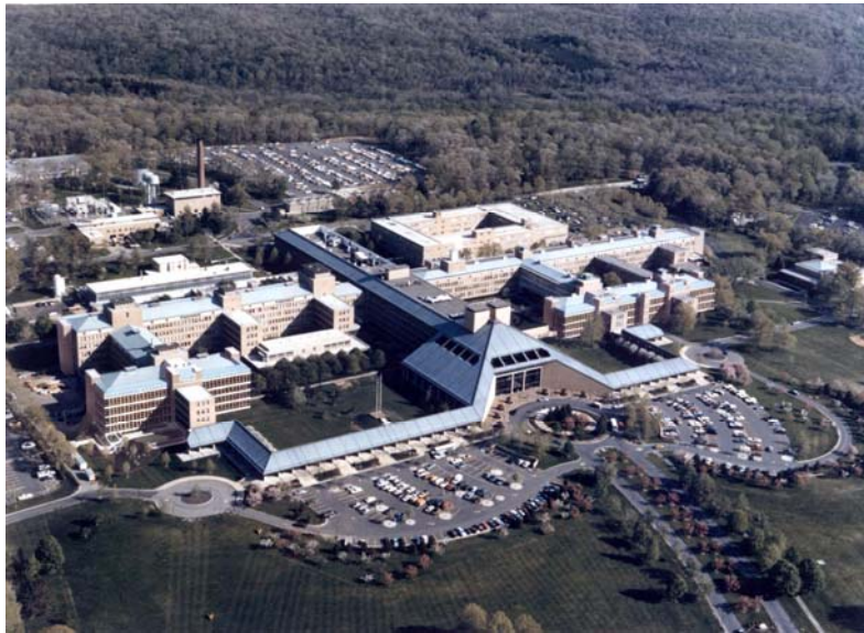
Fig. 2-5. Buildings 6 and 7 at Murray Hill were completed in 1974 and were situated between Buildings 1 and 2, replacing what used to be a Concourse. Building 7 was to the rear; Building 6 with its pyramid-like structure was to the front and became the main entrance to Bell Labs. Two covered walkways extended to the sides of the pyramid, like welcoming arms. Executive offices and the library were in the pyramid structure of Building 6. This dramatic aerial photograph is from the early 1980s. [Photo courtesy of Alcatel-Lucent USA Inc. / Bell Labs.]
