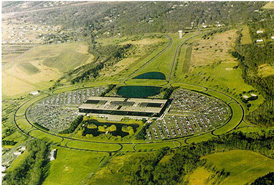
Fig. 4-1. Aerial photo of the Holmdel building, originally designed by Eero Saarinen, and the parking lots, roads, and ponds. The building was expanded in 1984. [Courtesy of the AT&T Archives and History Center.]
