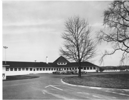
Fig. 4-6. Before the Saarinen building was constructed on the Holmdel property, a number of one-story buildings housed the Bell Labs researchers who worked there, mostly on antennas and radio waves. This photograph is from 1950, before these researchers were moved to a new building in Crawford Hill and the old Holmdel buildings razed. [Photo courtesy of Alcatel-Lucent USA Inc. / Bell Labs.]
