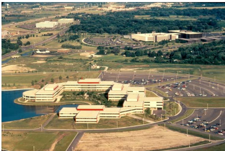
Fig. 4-9. Bell Labs R&D in switching was conducted at the Indian Hill, Illinois complex, consisting of many buildings, shown here in 1983. [Photo courtesy of Alcatel-Lucent USA Inc. / Bell Labs.]
