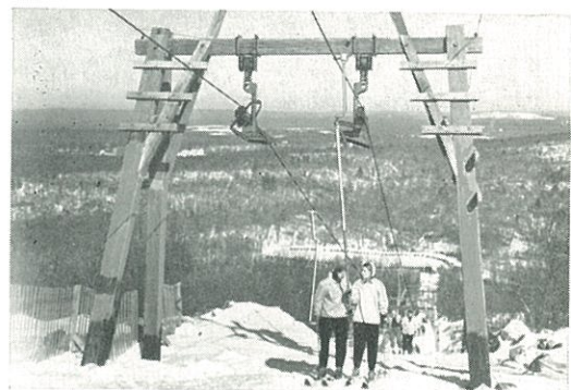
Telescoping Tube towing outfit for smooth slopes where snowfall is not extensive.
