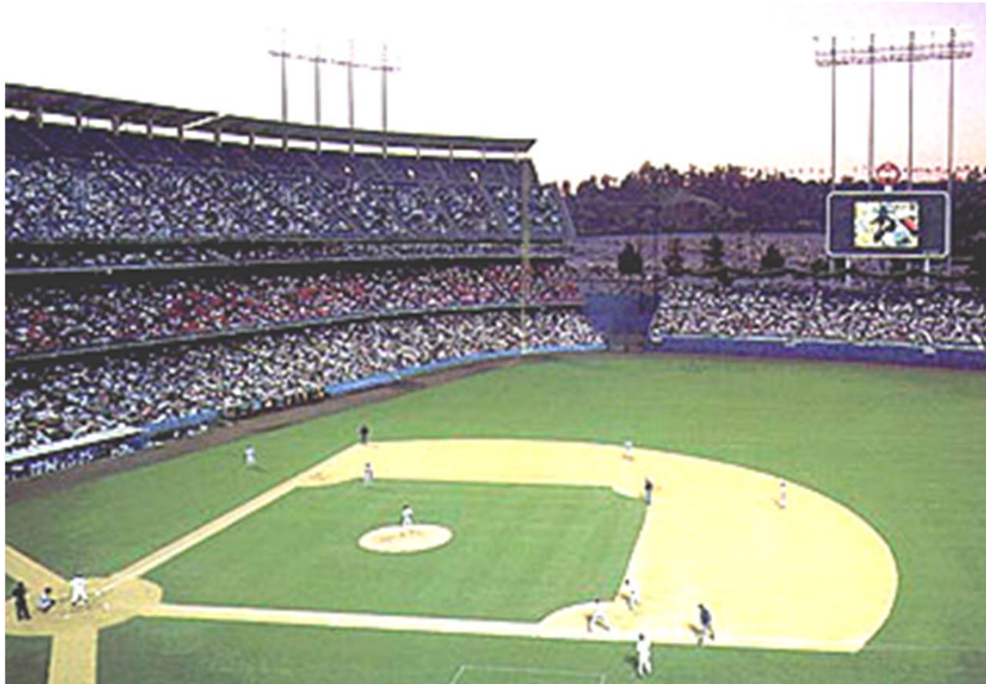
Large-scale color display system at Dodger Stadium
