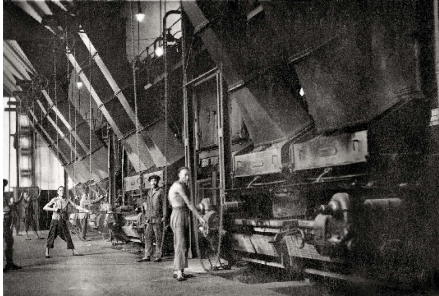
A view of the boiler house, 1920s Workers fuel the steam boilers in the boiler house of the company's power plant.
