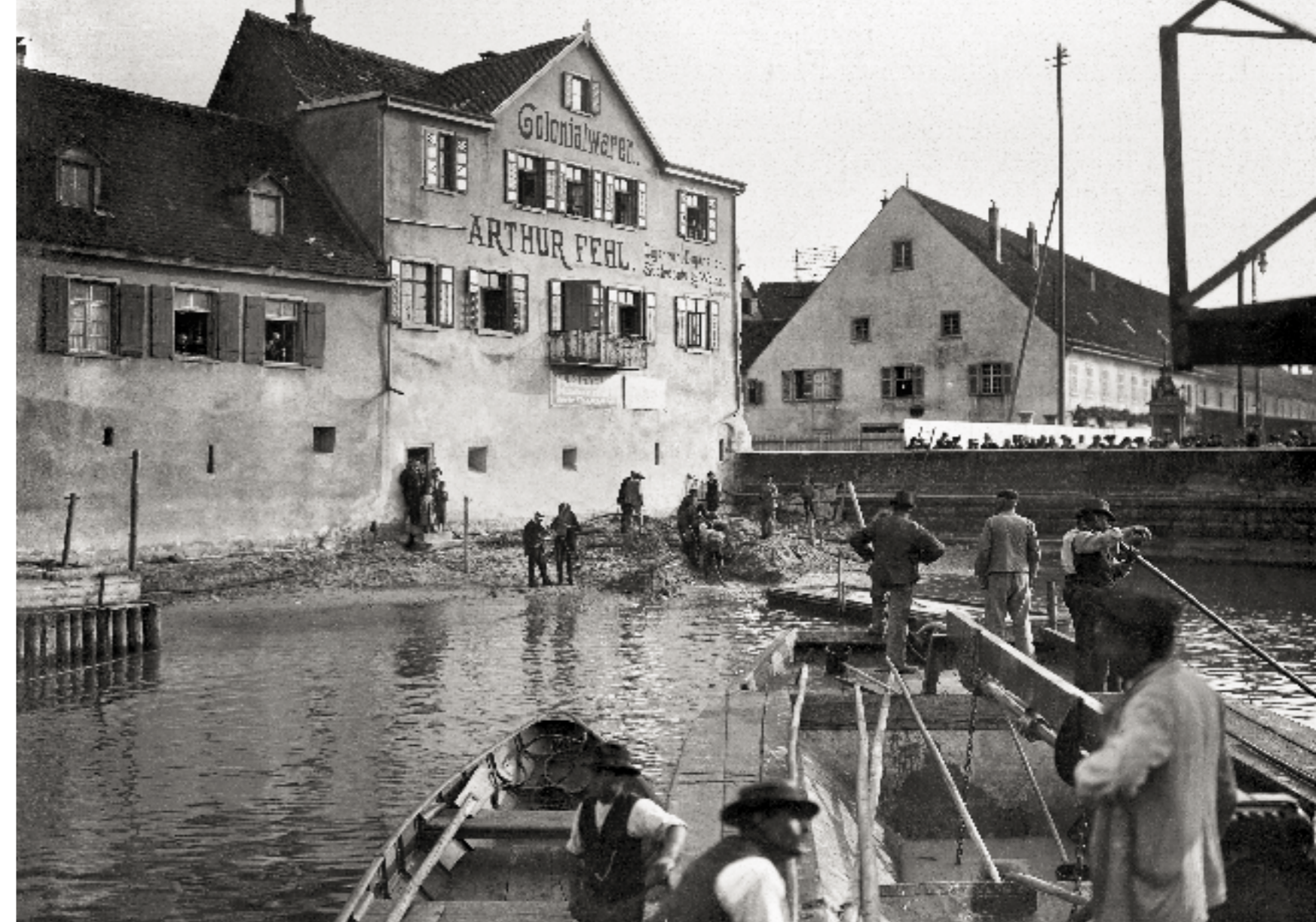
Laying the shore end of the cable in the dredged channel off Friedrichshafen, 1906
