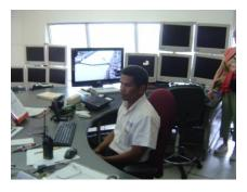
Four years ago, a computer control system was installed to replace the mechanical hand-operated lock system on the big table. Today, computer software issues the commands to the electrical system to perform the stream of activities to 'lock through' a ship. With the aid of computer surveillance, lock operators can keep track visually of all aspects of the ship and lock gate movements into the far corners. They can spot problems more easily and more quickly than could the manual system.
