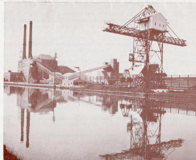
Will County Generating Station, Commonwealth Edison Company
