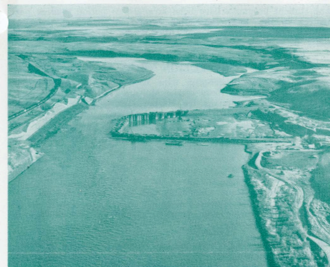
Cofferdam at Ice Harbor
