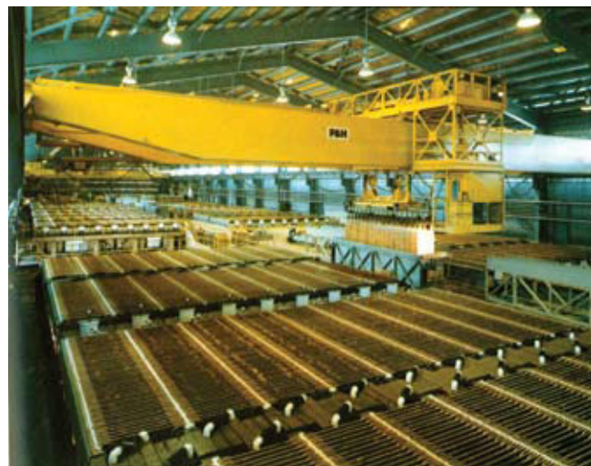
Anamax Mining Company’s copper recovery plant in Sahuarita, AZ, around 1980.
