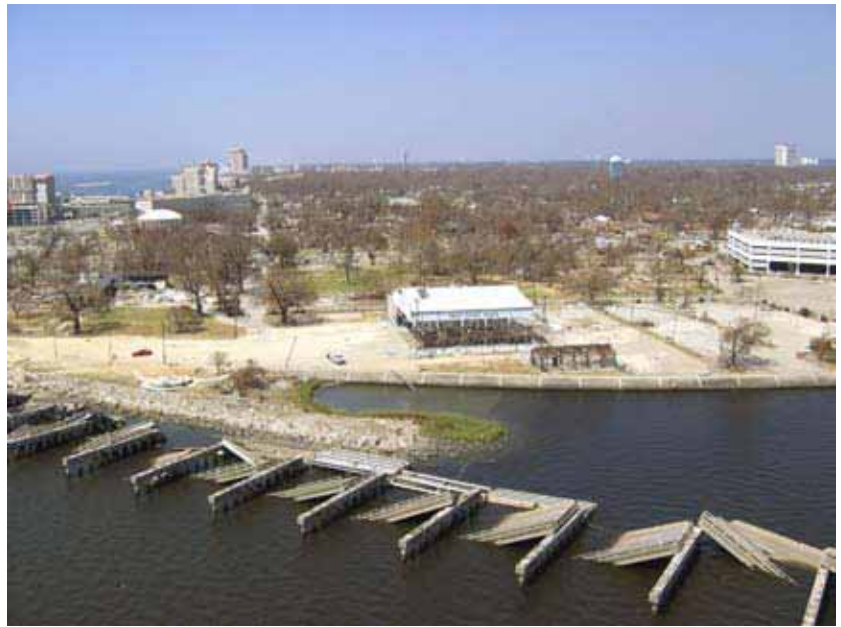
Figure 1. U.S. 90 Bridge in Biloxi, MS (Photo credit: NOAA)
