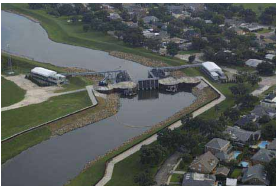
Figure 8. Orleans Avenue Canal (Photo Credit: US Army Corp of Engineers)
