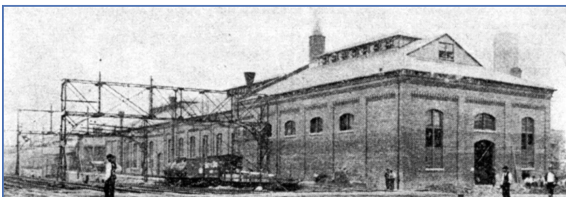
figure 2. Exterior view of the Camden generating station during construction, circa 1895 (source: 13 July 1895, The Electrical World , p. 54).
