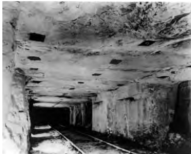
Roof bolts installed at the Isabella coal mine in 1949.
