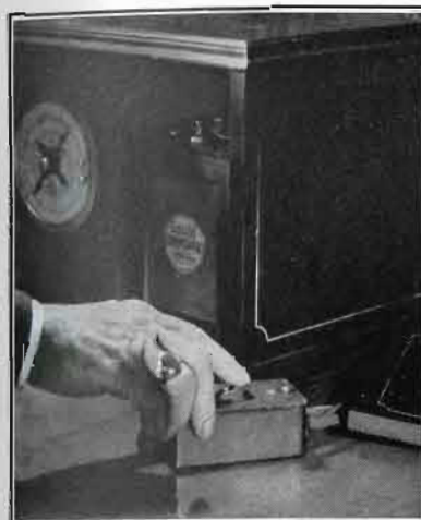
Cut Showing Use of Master Control Switch
