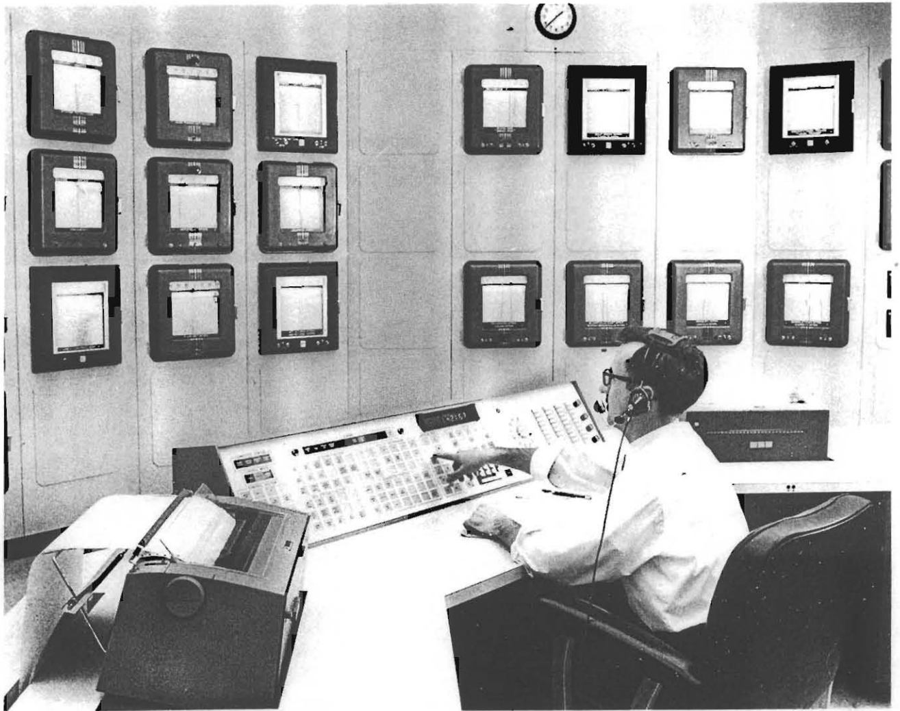
Dispatcher's console, printers, and meters at Allegheny Power System's dispatch center, Charleroi, Pennsylvania.
