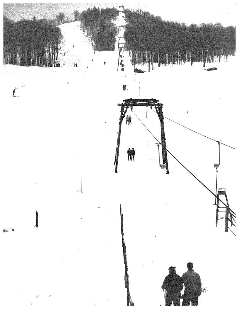
At Mount Tremblant there is a rise of 730 feet in a slope of 3428 feet, up which 450 skiers an hour can be transported at 8 minutes per trip. The Cannon Mountain Lift, which can accommodate 300 skiers per hour, takes 5 minutes to travel up the 2075 foot slope whose rise is 770 feet.
