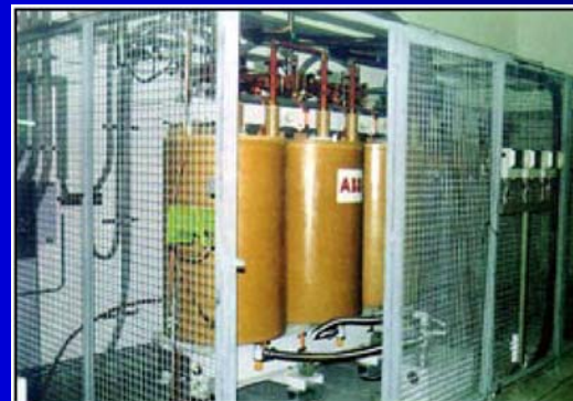
A 630-kVA demonstration HTS transformer resulting from an earlier ABB project. (ABB)
