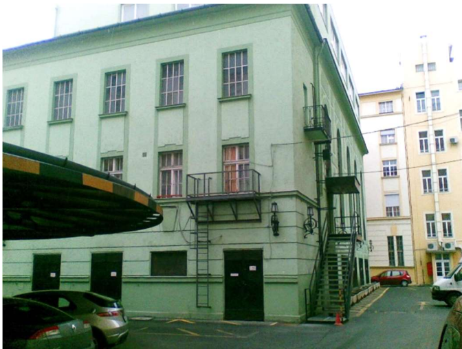
Fig. 21.: The old power house – today [17]
